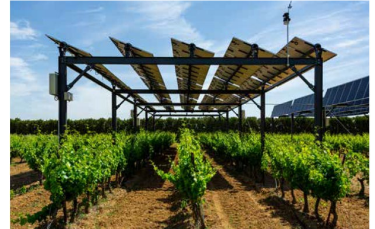
Agrivoltaics with solar tracking system in France.
