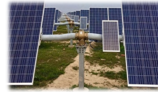
Decentralized: selfpower by auxiliary module
