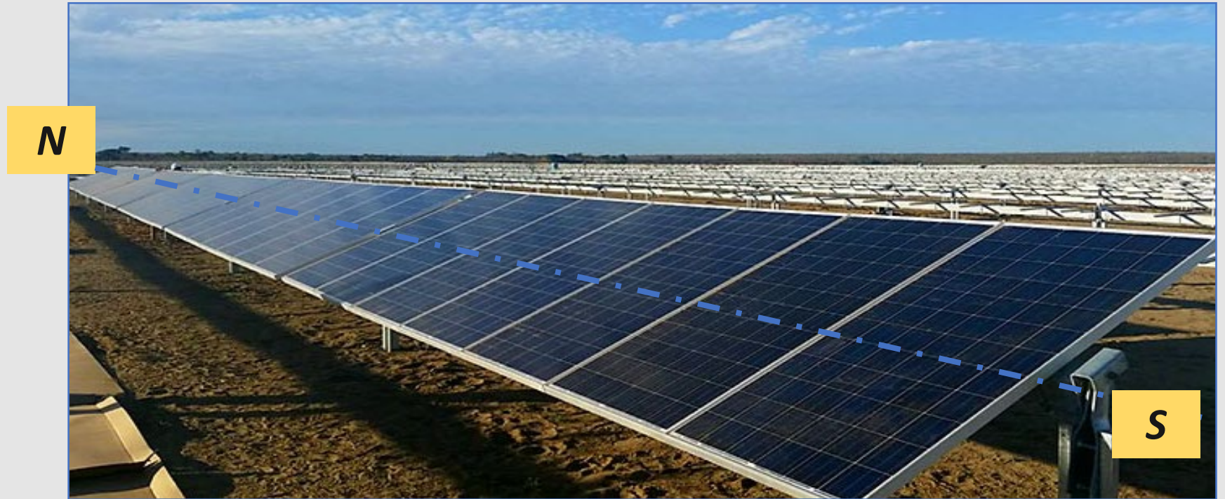
Horizontal single axis tracking: Rows of modules are usually orientated in a north-south line rotating from east to west.
