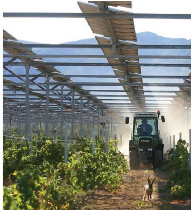
Dynamic shades Agri-PV system, viticulture.
