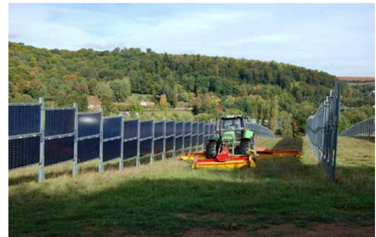
Vertically oriented bifacial modules in the Eppelborn-Dirmingen solar park, 87
