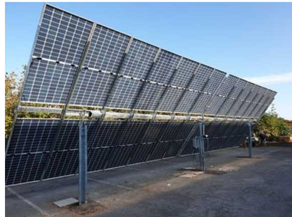
Figure 3 - HDG tracker structure, with the typical silver-grey colour.
